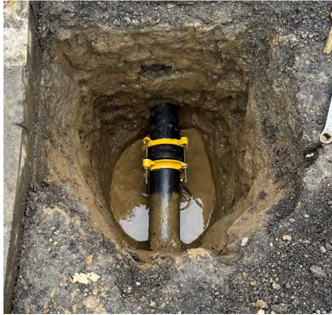
McLoughlin Main Break Repair
