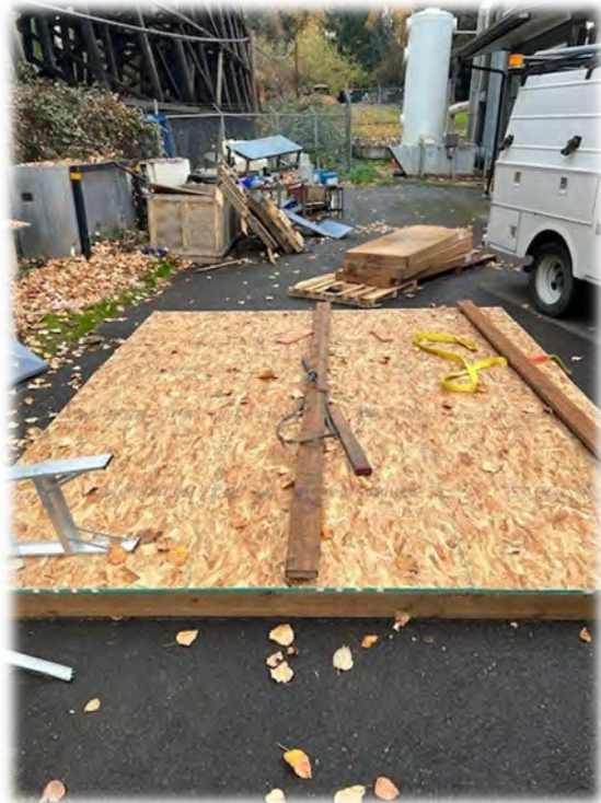
Flooring for New Material Storage
