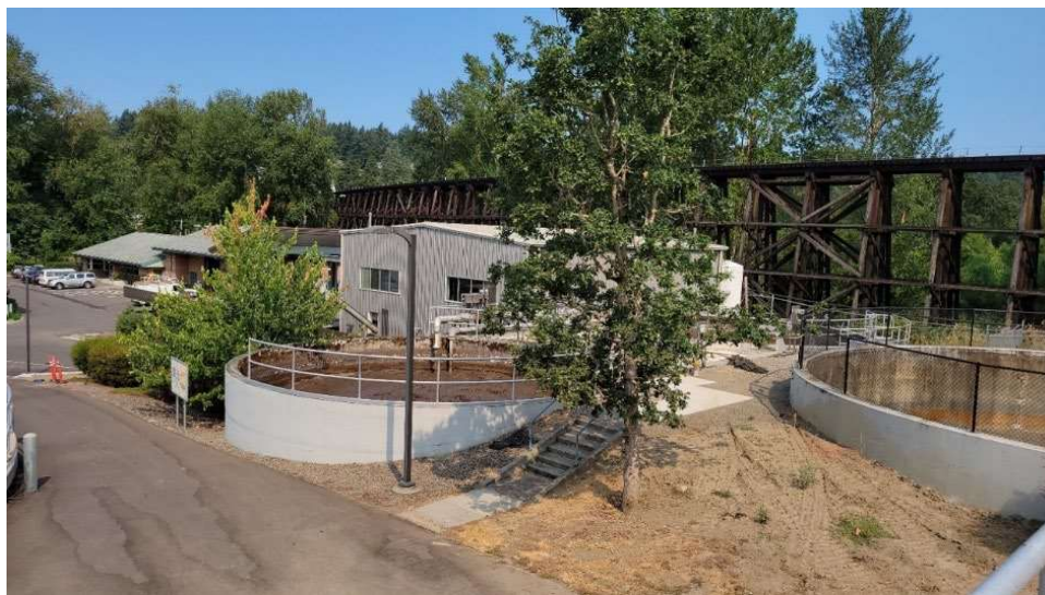
Figure 29. Circular aerobic digester
