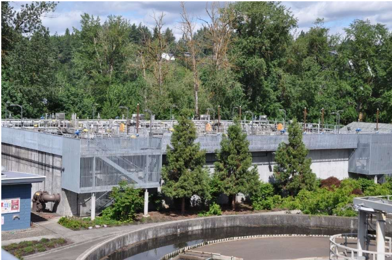
Figure 20. Aeration basin structure
