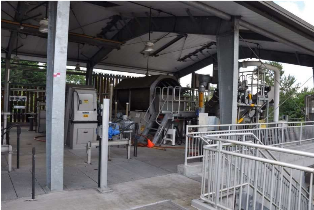
Figure 13. Mixed liquor rotary drum screen
