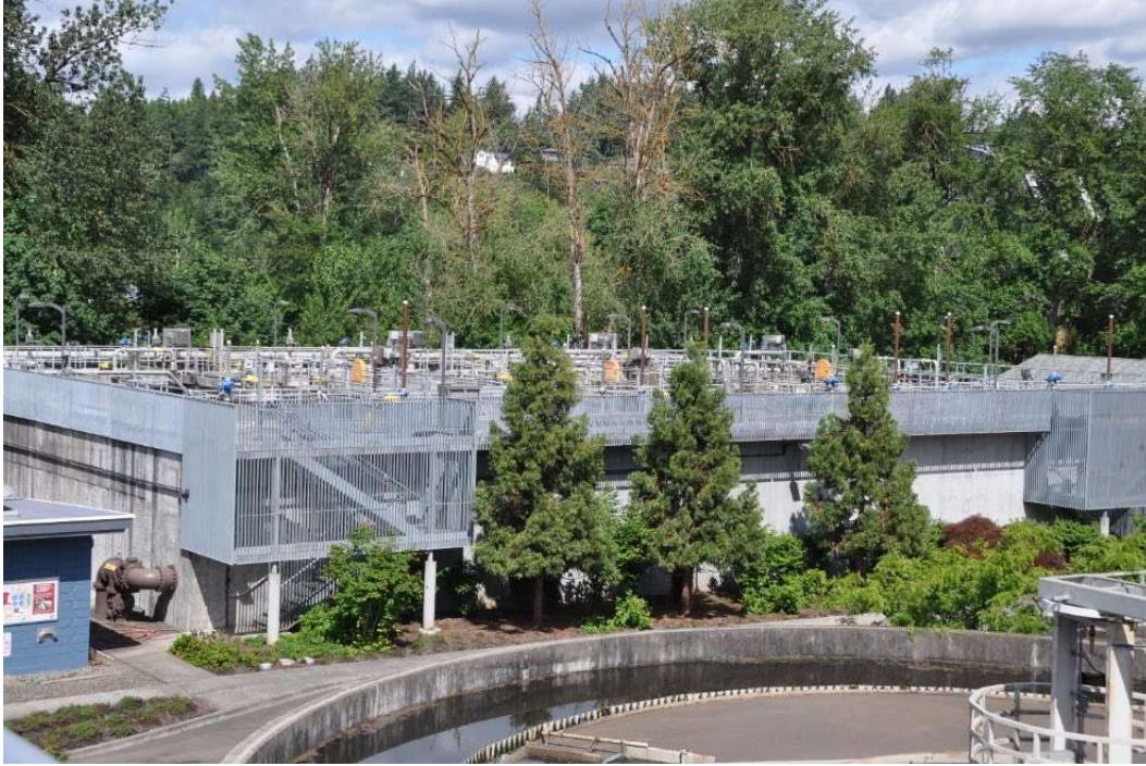
Figure 15. Aeration basin structure
