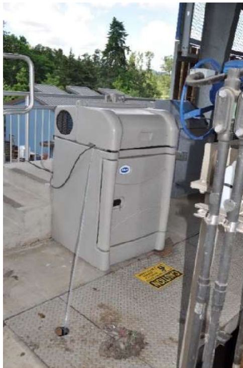
Figure 8. Influent composite sampler
