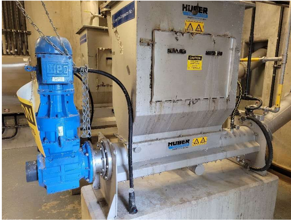
Figure 15. Screenings washer/compactor side view
