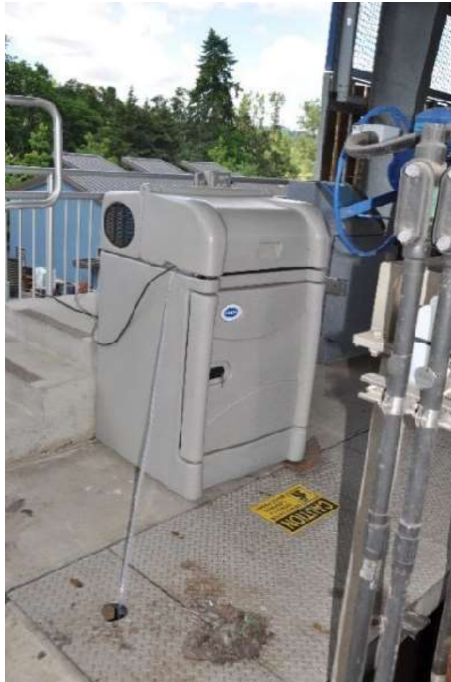
Figure 9. Influent composite sampler
