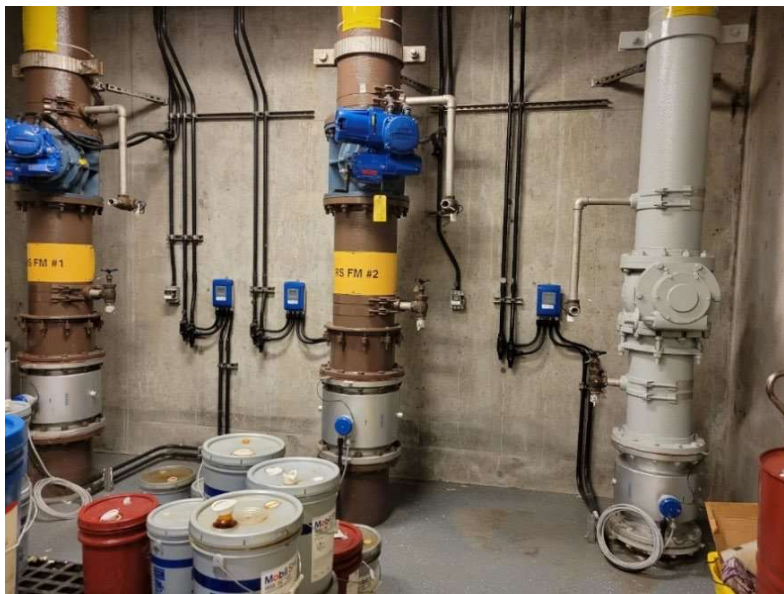
Figure 6. Influent pump and plant drain pump force mains
