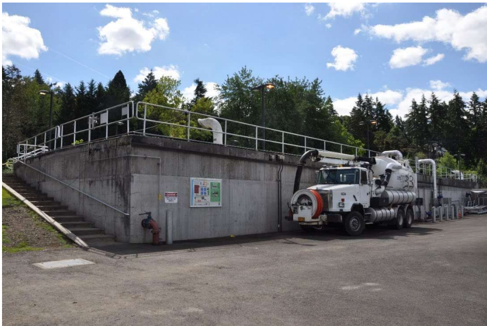
Figure 37. Aerobic Digesters 1 and 2 from below
