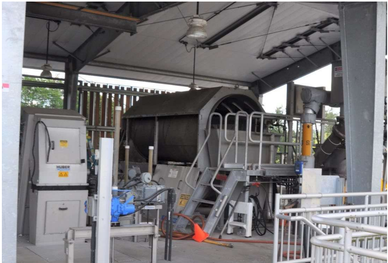
Figure 16. Mixed liquor rotary drum screen
