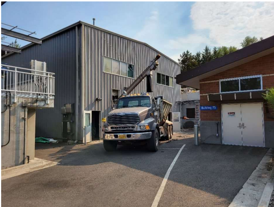
Figure 46. Truck loadout at Solids Handling Building
