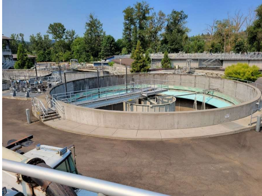
Figure 22. Original secondary clarifier
