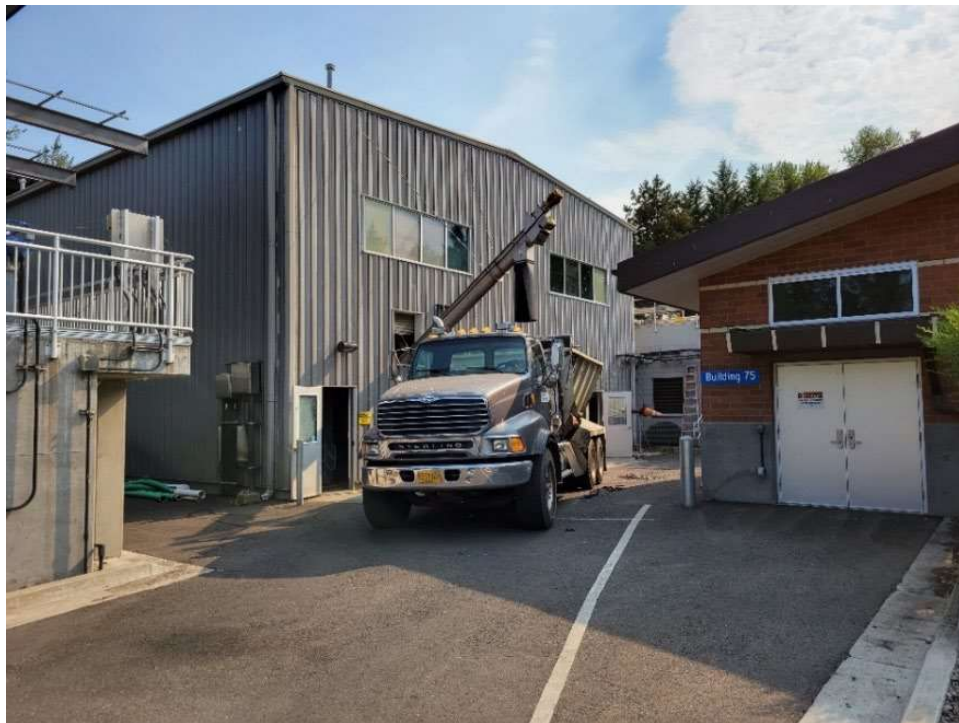
Figure 33. Truck loadout at Solids Handling Building
