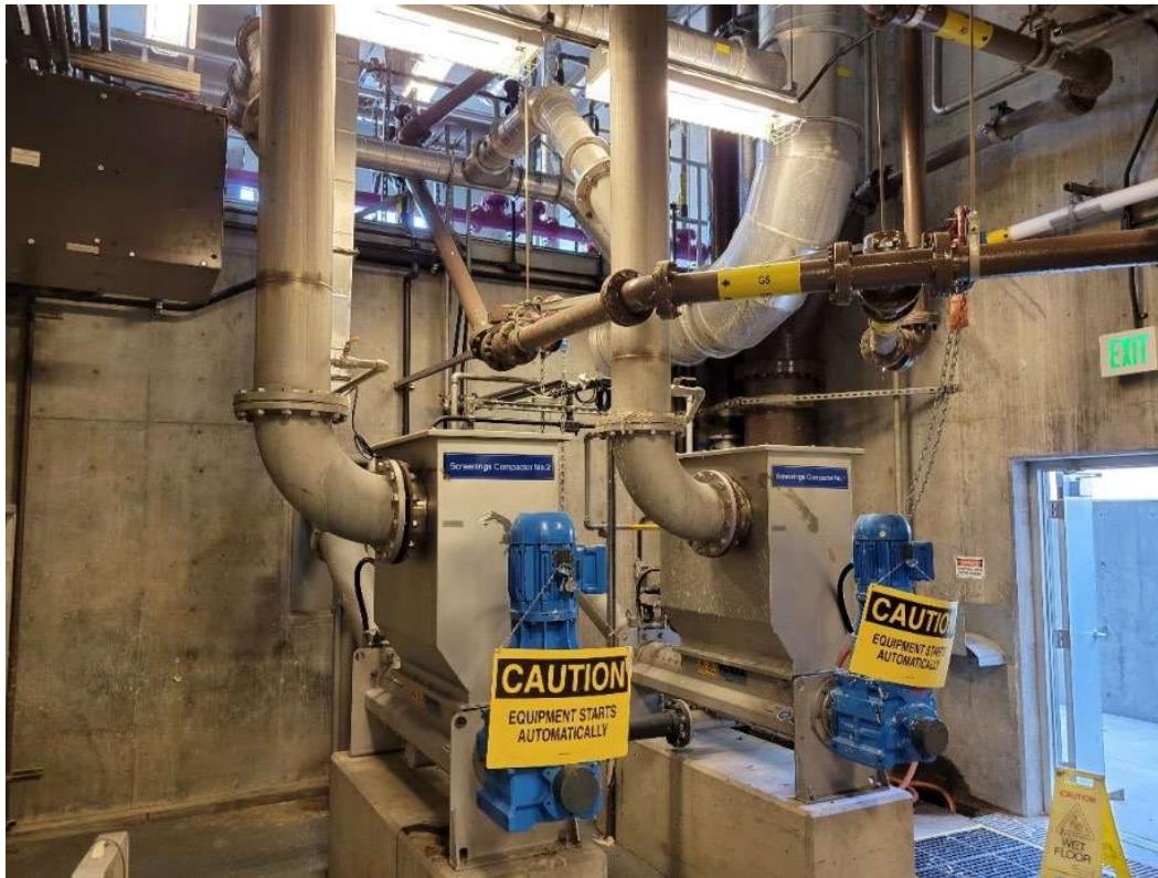
Figure 12. Screenings washer/compactors
