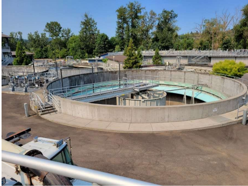
Figure 29. Original secondary clarifier
