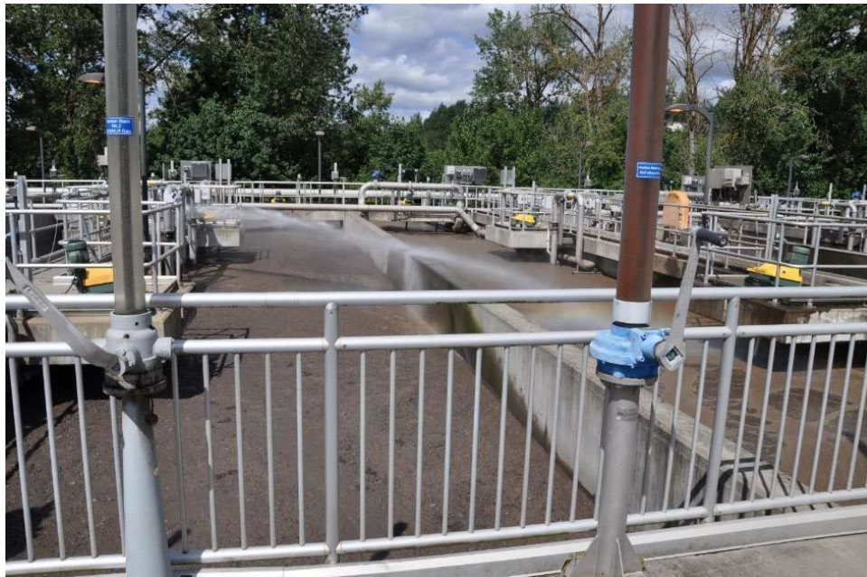
Figure 17. Aeration basin showing use of hoses for spray water
