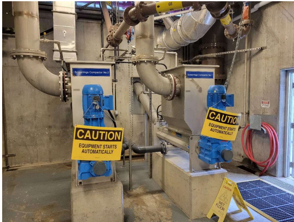
Figure 14. Screenings washer/compactors
