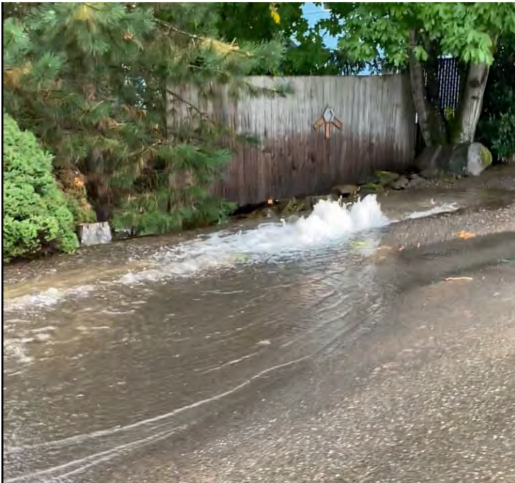
Photo 7: Main leak on Hull
