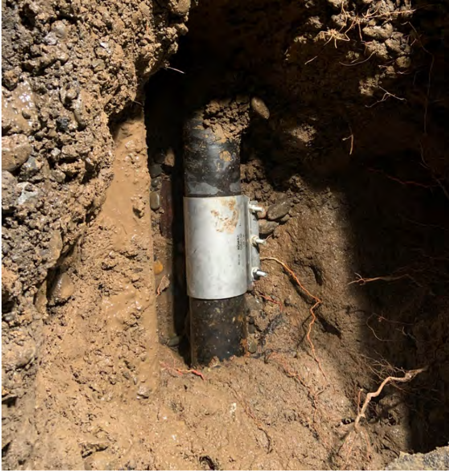
Photo 9: Water main repair on Vineyard
