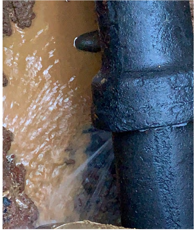
Photo 6: Bell-joint leak on Oatfield
