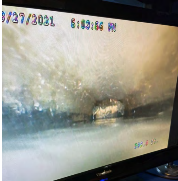
Photo 1: Sewer lateral camera view
