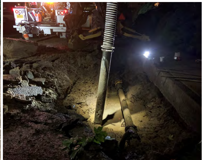
Photo 8: Water main repair
