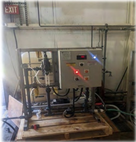
Temporary polymer skid.
