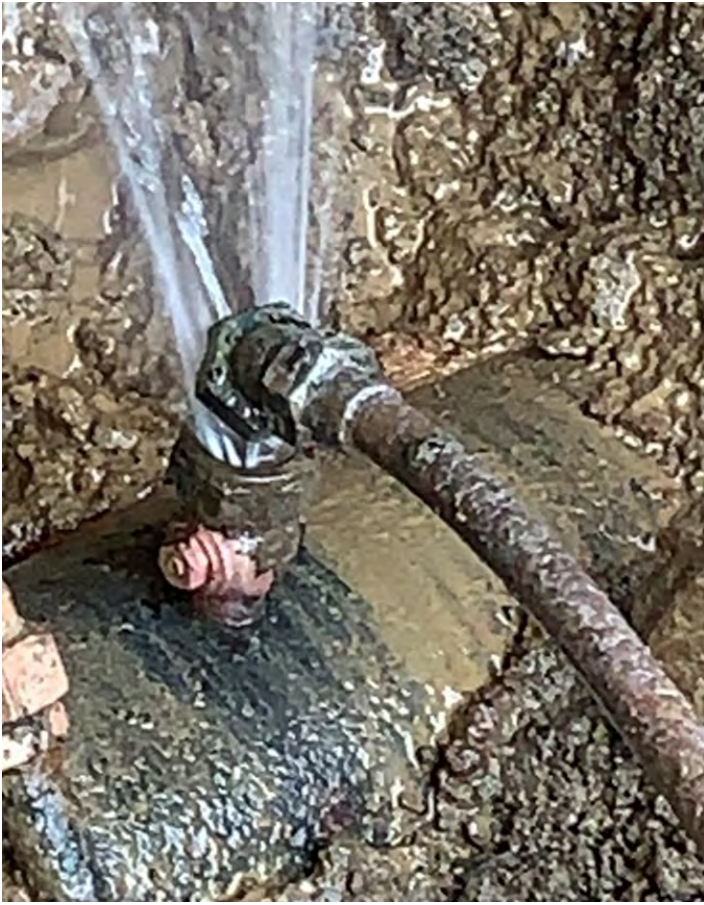
Photo 5: Service leak on Aldercrest
