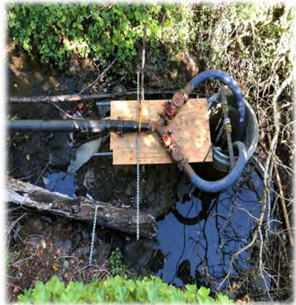
Temporary pump around installed.
