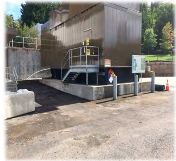
Scrap Pile all cleaned up!
