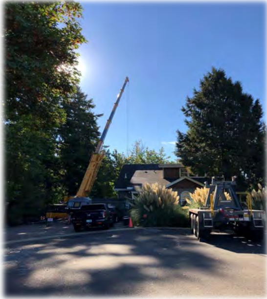
Crane lifting equipment into place PS#5.
