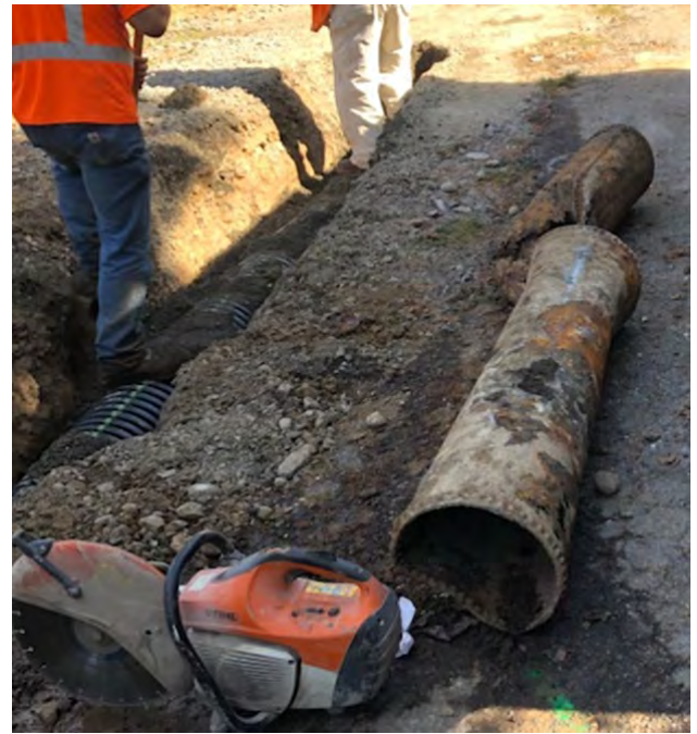
Photo 4: Old stormwater "pipe"
