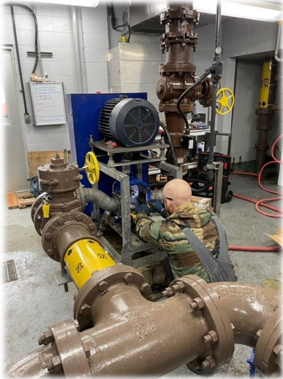
Mechanic Abe Merritt Swapping Lobes on Pump.
