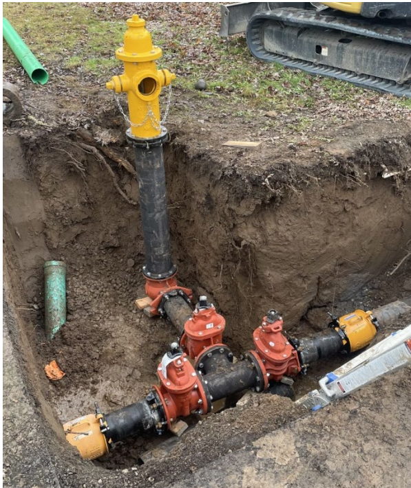
SE Risley Hydrant Replacement
