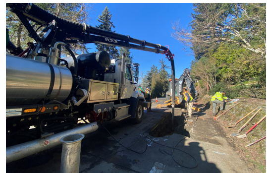
Image: Vactor truck repairing a leak on SE Oatfield Rd.
