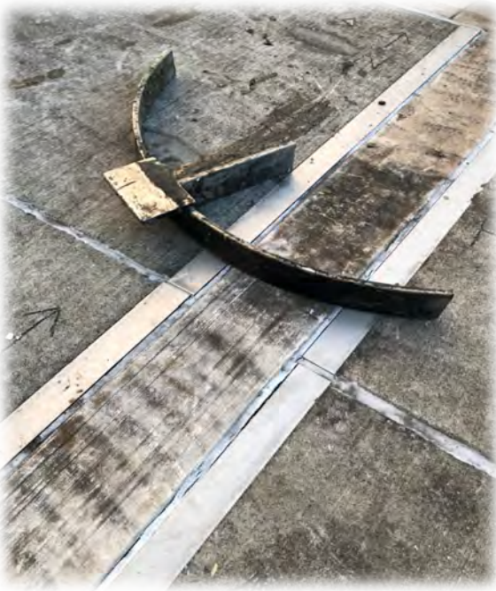
7) Cross bar cut and removed
