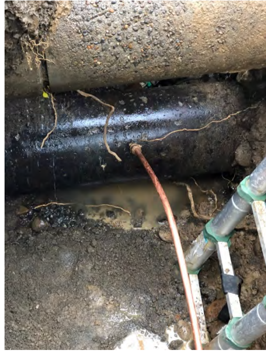
NEW SERVICE ON 16" MAIN
