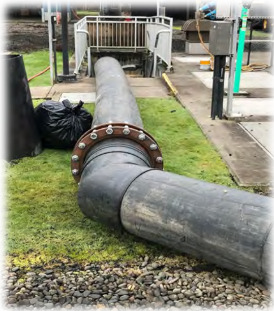
1) Pipe from the pump station
