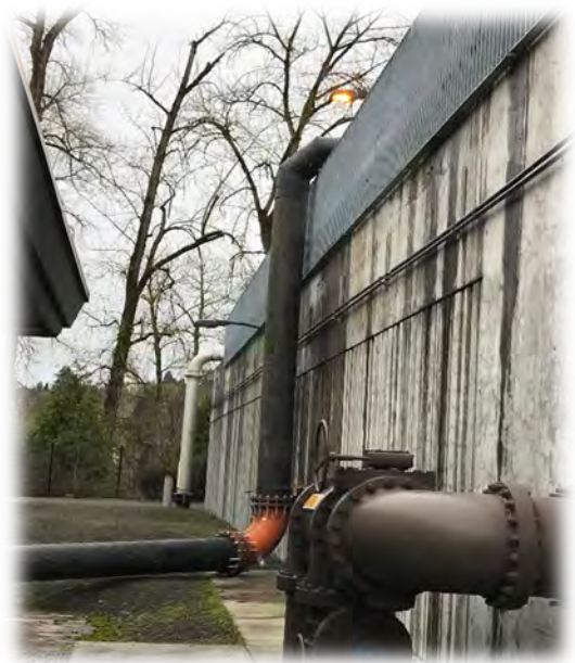
2) Pipe up to the aeration basin
