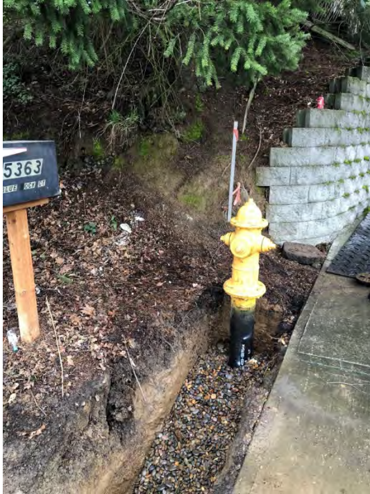
NEW HYDRANT INSTALL ON OATFIELD
