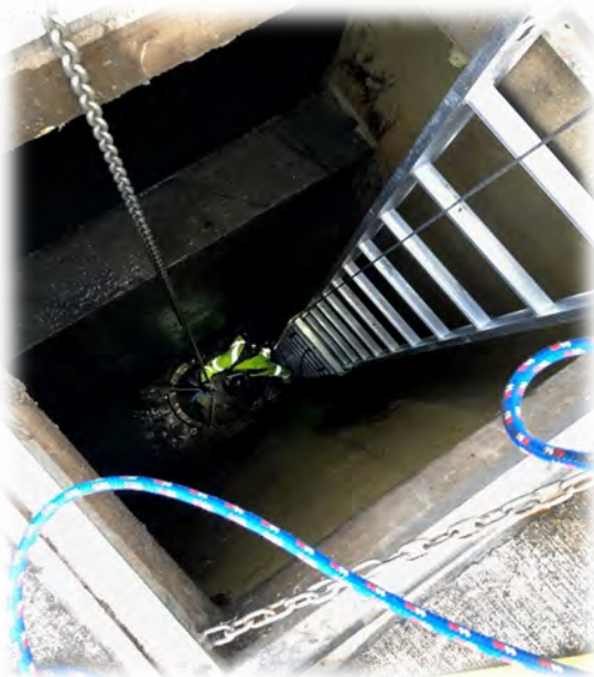
3) Entry to the wet well
