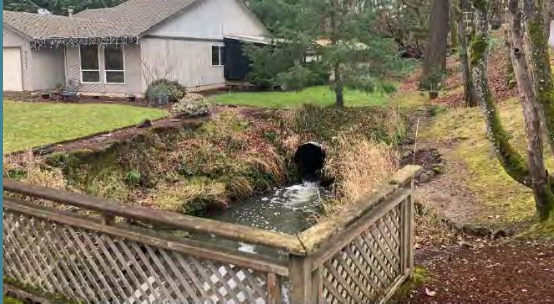
Figure 65. Culvert upstream of SE Walta Vista Rd that is presumed impassable for fish (culvert extends upstream through SE River Road in background of photo, culvert length is an estimated 80 or more meters).
