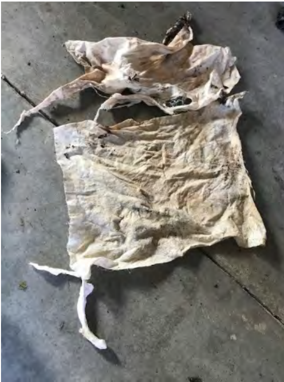
RAGS PULLED FROM SEWER MAIN
