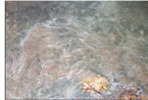
Sporolitis filamentous bacteria, also known as “sewage fungus” can be used to track down sanitary sewer leaks.
