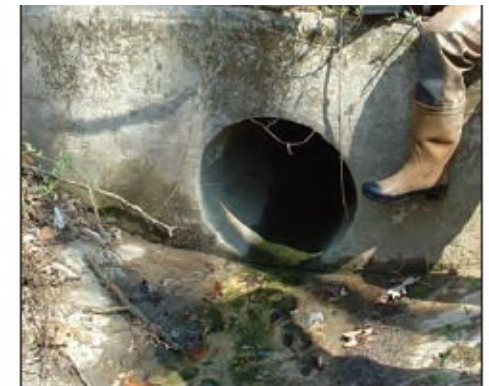
The drainage to this outfall most likely has a high nutrient concentration. The cause may be an illicit discharge, but may be excessive use of lawn chemicals.
