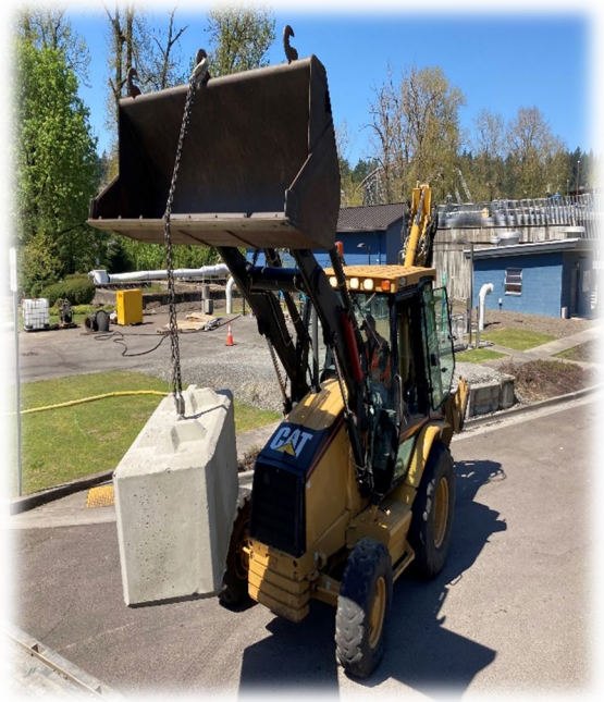
6) Ultra blocks for biosolids storage
