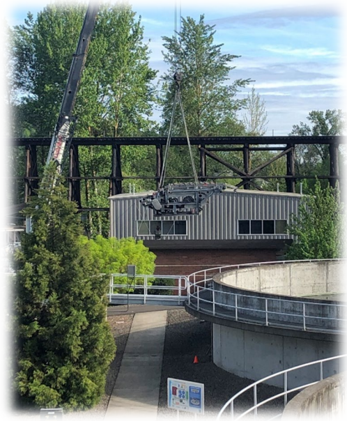
2) Belt Press #2 on the way back
