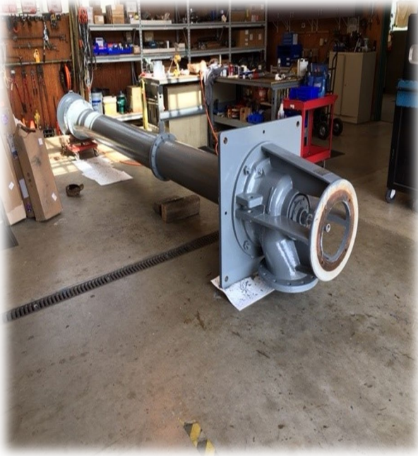
5) Mixed Liquor Pump #3 all rebuilt
