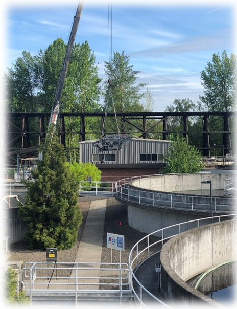
1) Belt Press #2 being lifted
