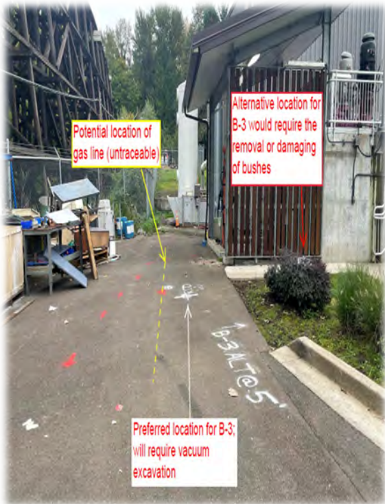
Overview of Geotechnical Location.
