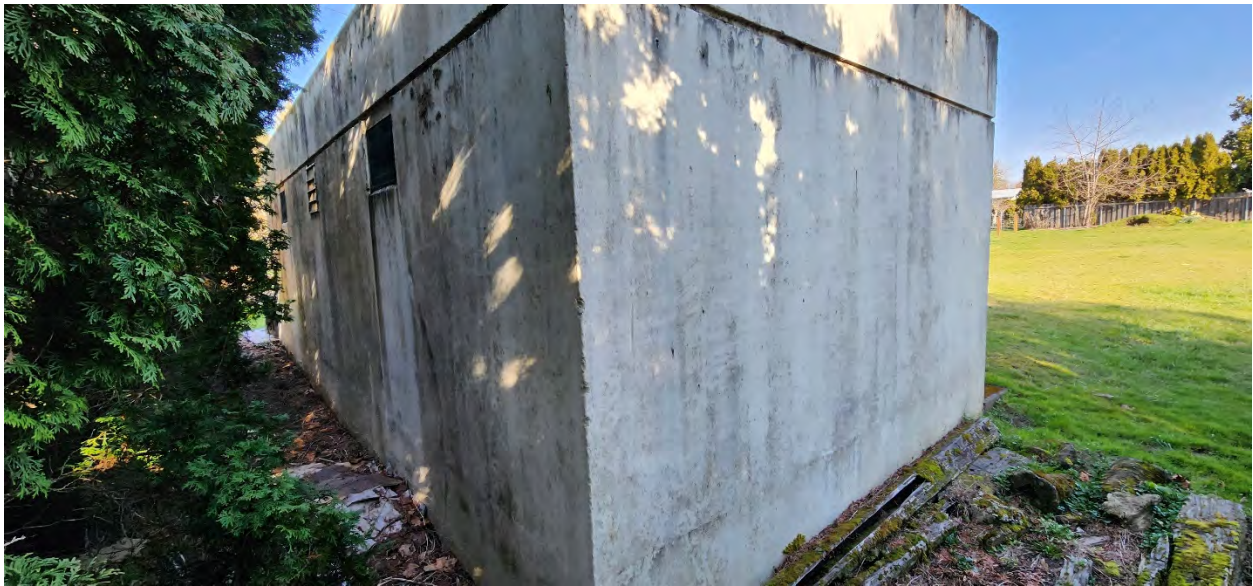
Figure F.2 - Southeast Corner of Pump Station
