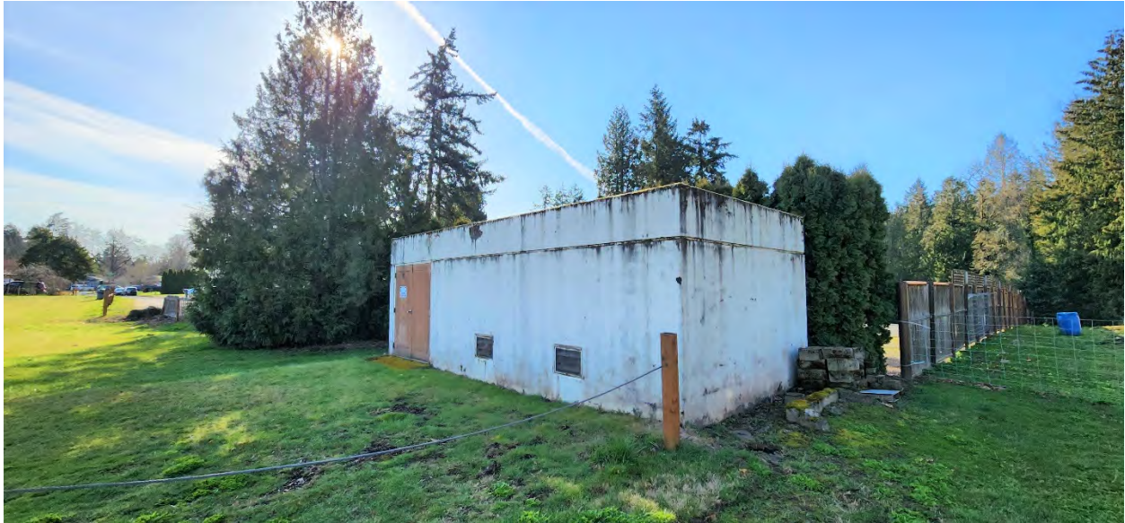
Figure F.1 - Northwest Corner of Pump Station
