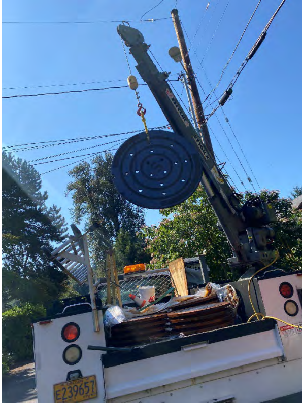
Removal of Storm Lid
