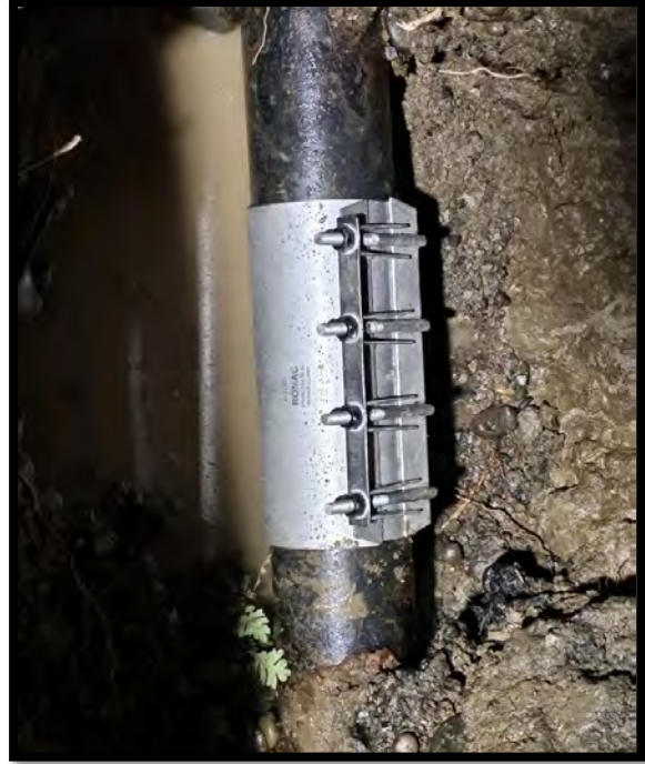
Westview Avenue Pipe Repair
