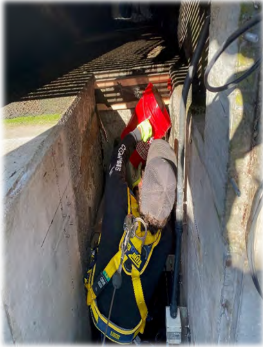
Effluent UV gate pad being poured.
