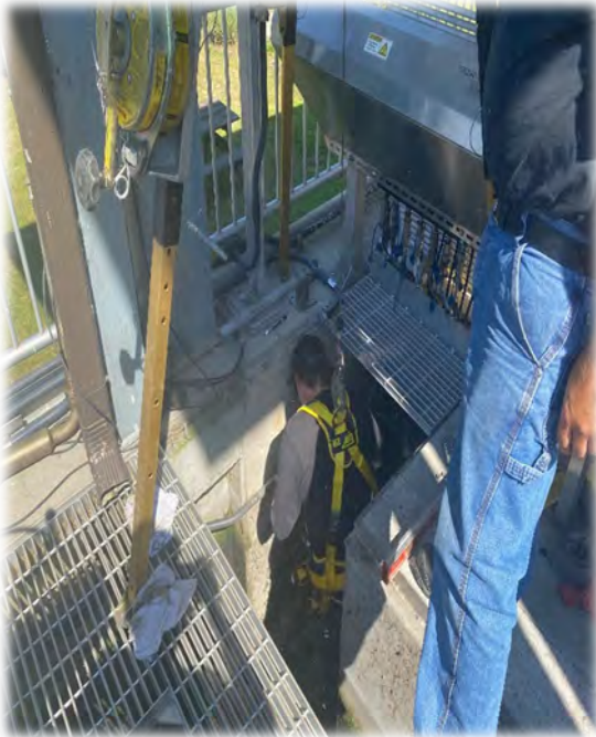
Conduit being relocated for UV gate.
