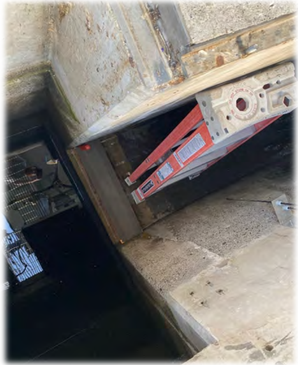
Effluent UV gate pad finished.
