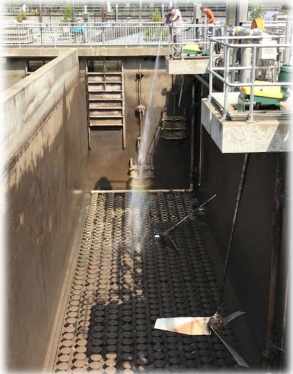
Photo 3 Aeration Basin #2 with blades at bottom
