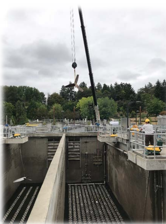
Photo 4 Crane removing blade and shaft
