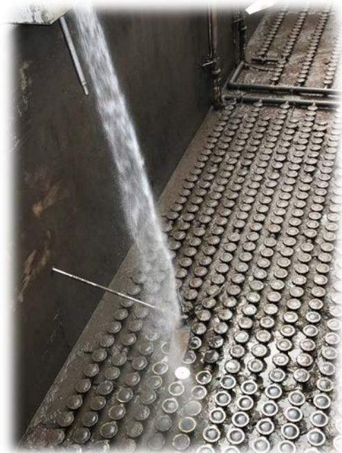
Photo 8 Another view of Aeration Basin #2
