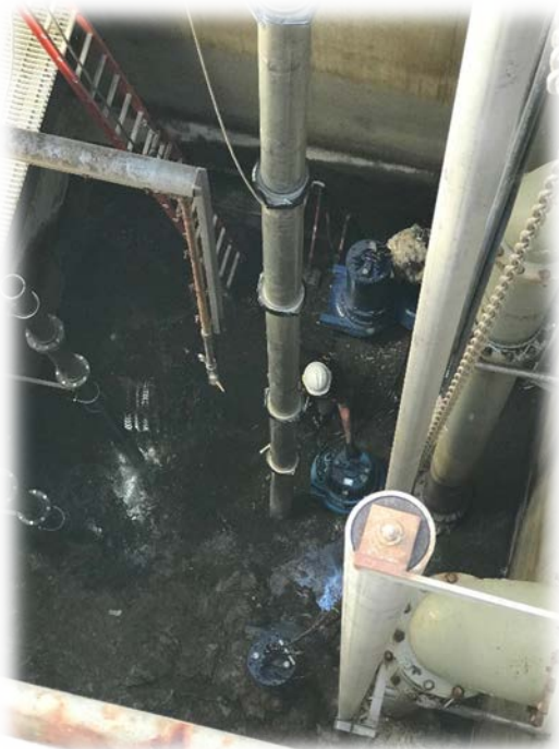
Photo 7 Wet well almost cleaned
