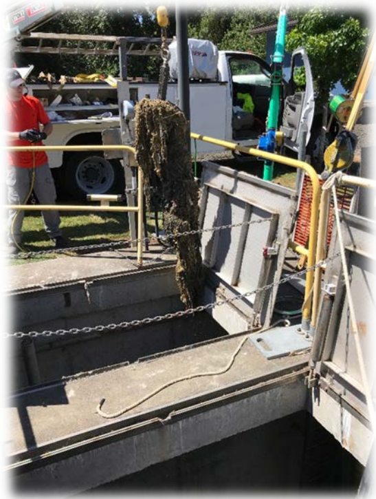
Photo 6 Debris removed from Pump Station #1
