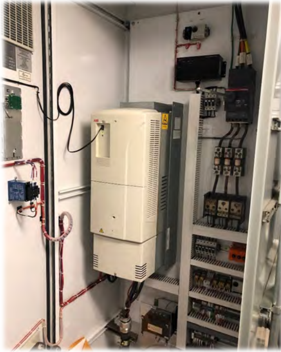
Variable Frequency Drive for IPS #1
