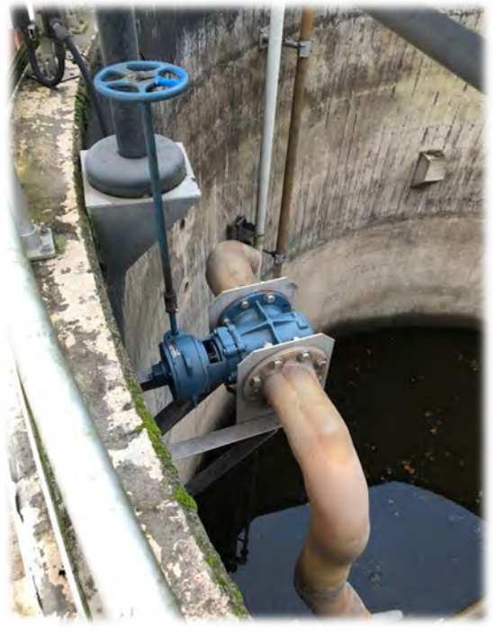
East RAS Pump Installation
