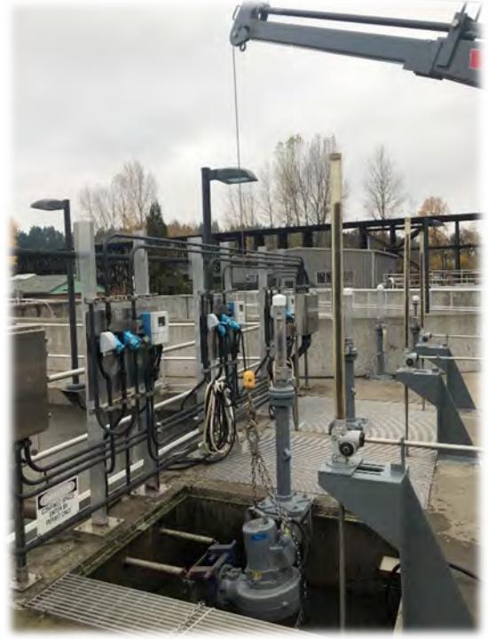
East RAS Pump Installation
