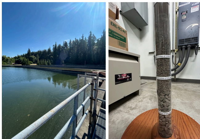
Slow sand filtration beds at the NCCWC treatment plant (left), and a representation of layers beneath the surface (right).
